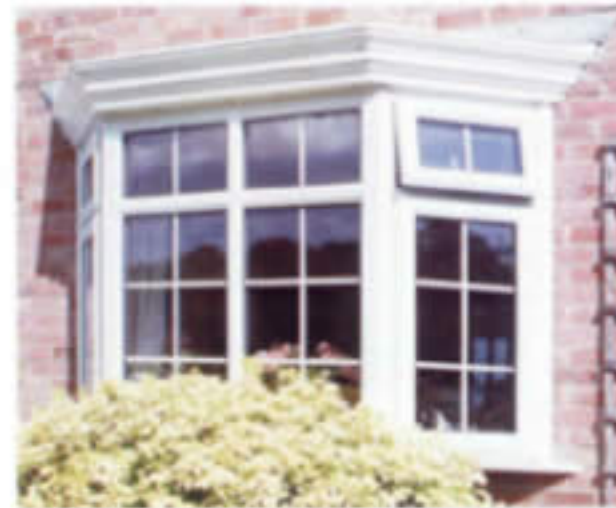
Bow Bay with GRP roof and Georgian Bars
